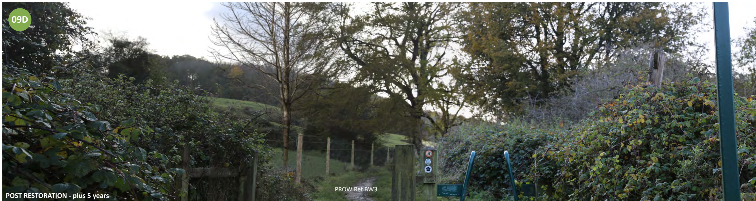
Photomontage Location 09. View looking south westwards from PROW ref. BW3, towards the proposed conveyor corridor and crossing point. Short range visibility (transient) of the elevated conveyor crossing point and surface level vehicular crossing. Associated fencing / gates and surfacing changes, with the existing PROW route travelling beneath the conveyor bridge. Native tree planting visible upon restoration, post the removal of the conveyor infrastructure.
