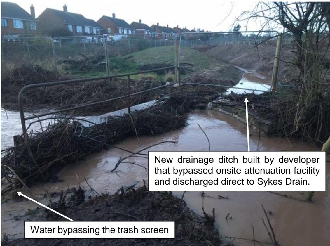
**Photo 5. (Sunday 16<sup>th</sup> February) showing the trash screen upstream of the culvert to be completely blocked to the extent that water is bypassing the screen on the left-hand side and the additional drainage ditch.**
