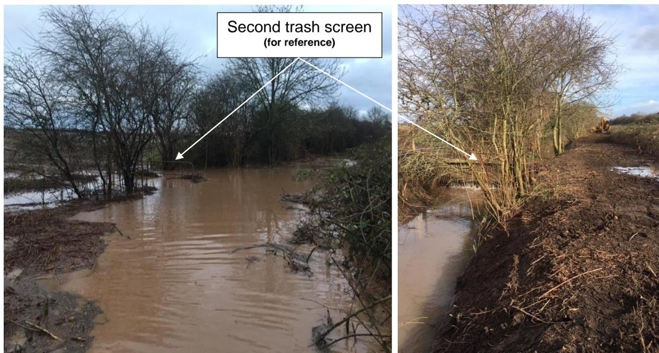
**Photo 2. (left) Sykes Drain looking upstream from boundary of 87 Clumber Drive showing surcharge on Sunday 16<sup>th</sup> February and Photo 3. (right) after trash screens and banks of watercourse cleared on Monday 17<sup>th</sup> February.**
