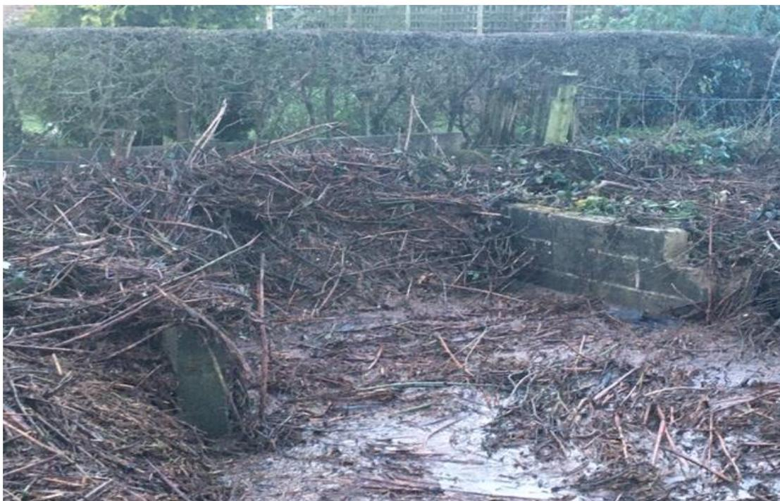
**Photo 6. (Sunday 16<sup>th</sup> February.) showing the debris blocking the trash screen on the mouth of the culvert. The trash screen is not visible due to the amount of debris.**
