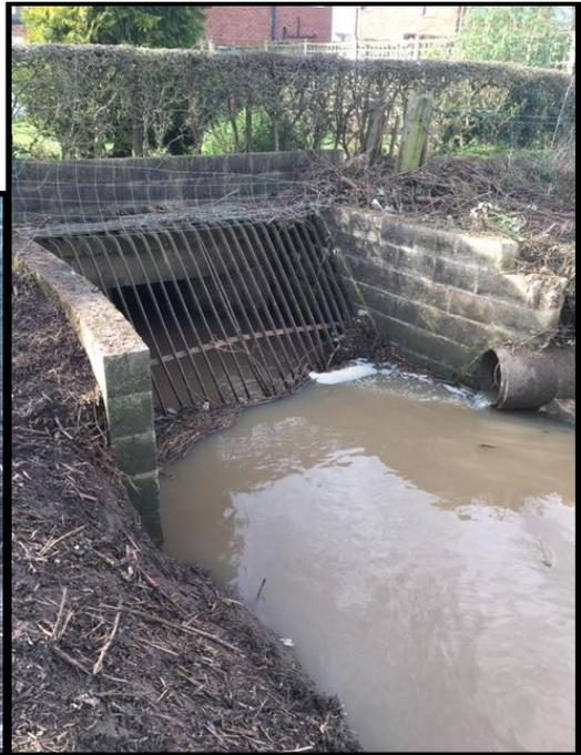
**Photos 7. (left) and 8. (right) of the trashscreen on mouth of culvert.**
