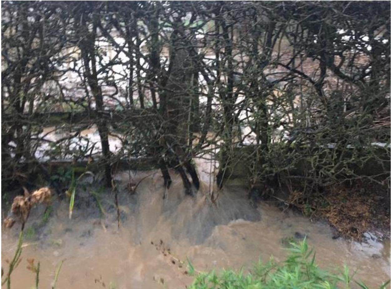
**Photo 4. taken at 0730 on Sunday 16<sup>th</sup> February from the garden of 87 Clumber Drive and showing water still flowing over the boundary from the surcharged Sykes drain.**
