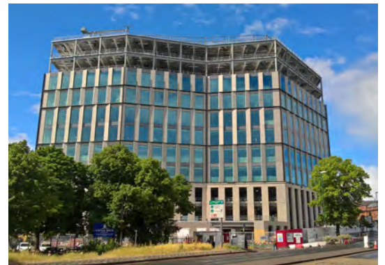
Inland Revenue building, Nottingham
