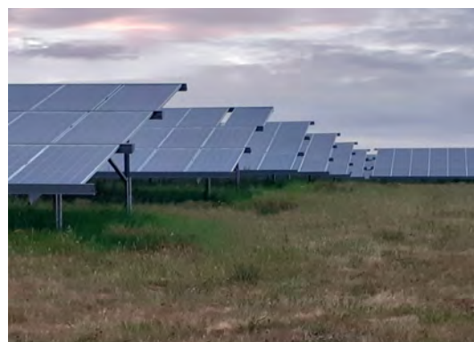
Solar Farm at Gedling Country Park
