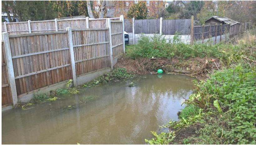
**Figure 7. Evidence of dyke backing up where it passes under an access road**
