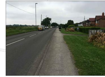
Existing footway to be widened to accommodate shared use cycle footway. Min. width 3.0m. Lighting columns to be relocated to the proposed back of footway.
