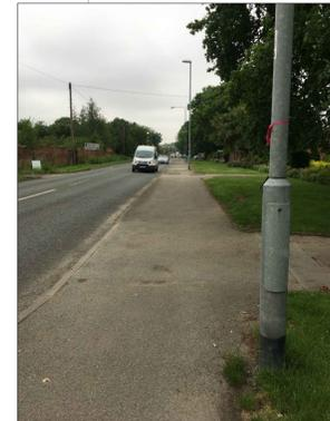
Existing footway to be widened to accommodate shared use cycle footway. Min. width 2.5m. Lighting columns to be relocated to the proposed back of footway.
