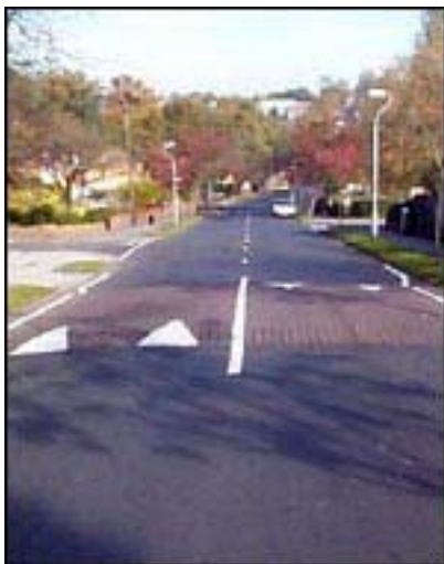
Fig 2 Flat top road hump incorporating block paving.
