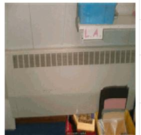
Presumed crocidolite asbestos. No access. Presumed to contai n Insulation board and gaskets
