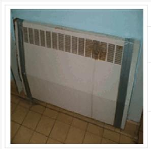
Presumed crocidolite asbestos. No access. Presumed to contai n Insulation board and gaskets
