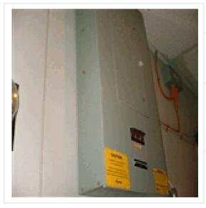
Presumed crocidolite asbestos. Presume to contain Insulation board, rope seals and flash pads
