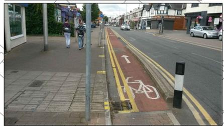
Footway widening to 3.0m to create shared use cycleway with full width resurfacing of footway. Tree canopies will need to be raised on Broxtowe Borough Council public open space
