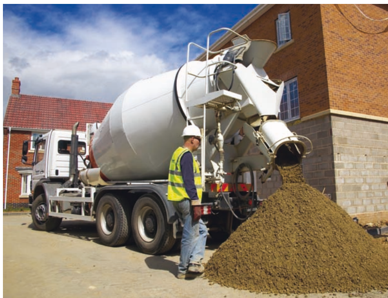
Image courtesy of Hanson Heidelberg Cement Group
