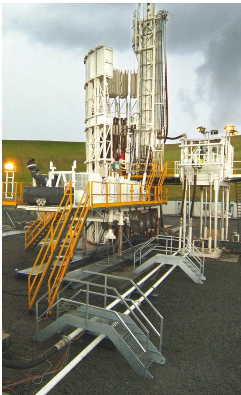
Coal Bed Methane drilling rig Image courtesy of Dart Energy (Europe) limited
