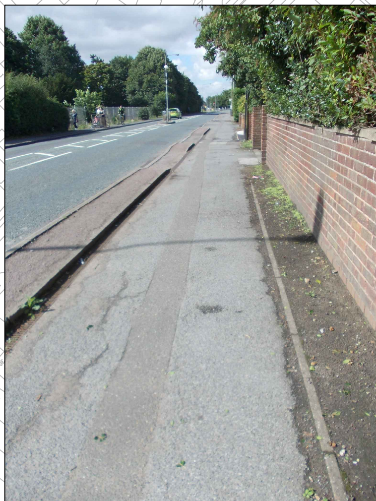
Existing footway edging to be replaced with splayed kerb.
