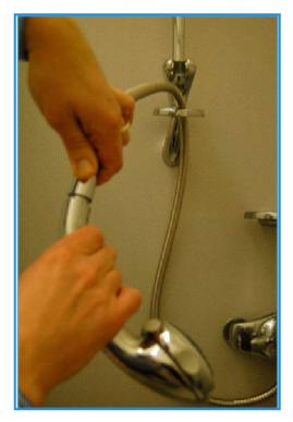
This shower has a restraining bar were the pipe is held. It may be necessary to remove the shower head before flushing.
