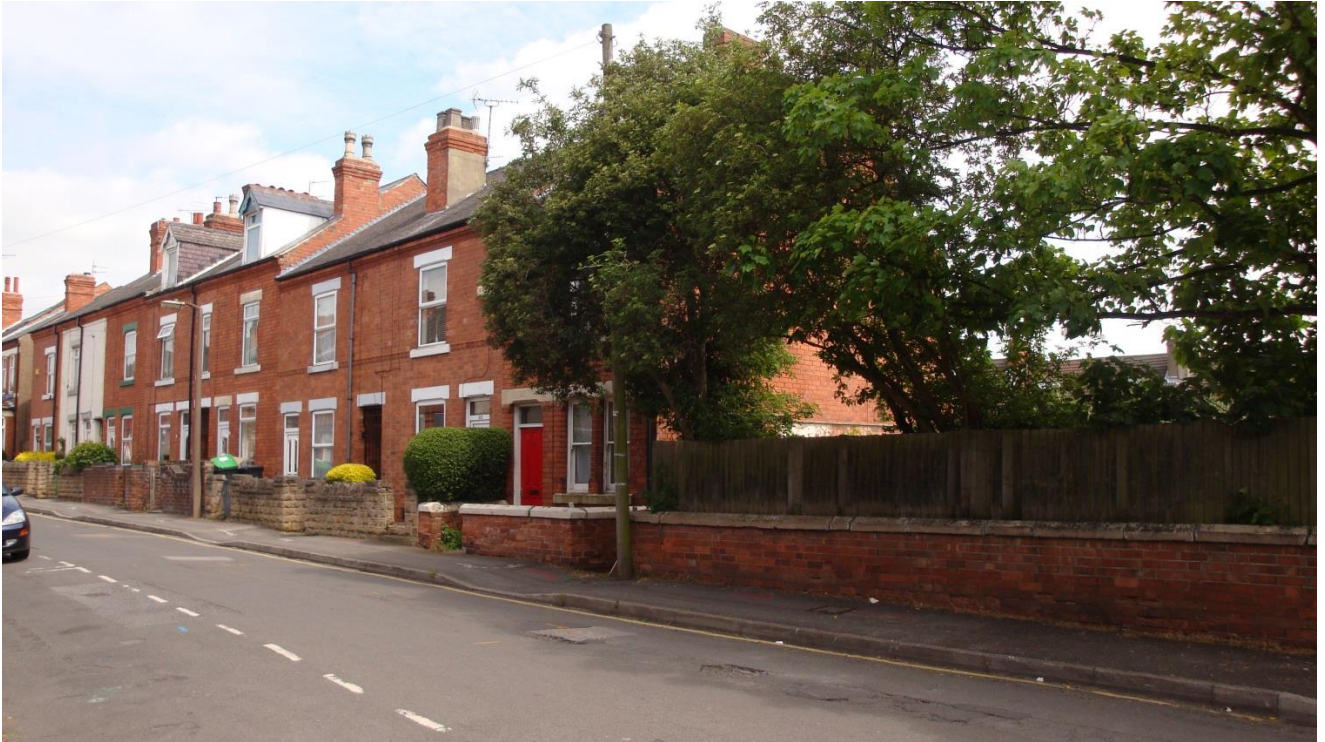
Figure B.3: West and south façade of 28 Titchfield Street (Ref: 4) and no. 28, 30, 32, 34 and 36 Titchfield Street to north of No. 28 (Ref: 1362, 1361, 1360 and 1359)
