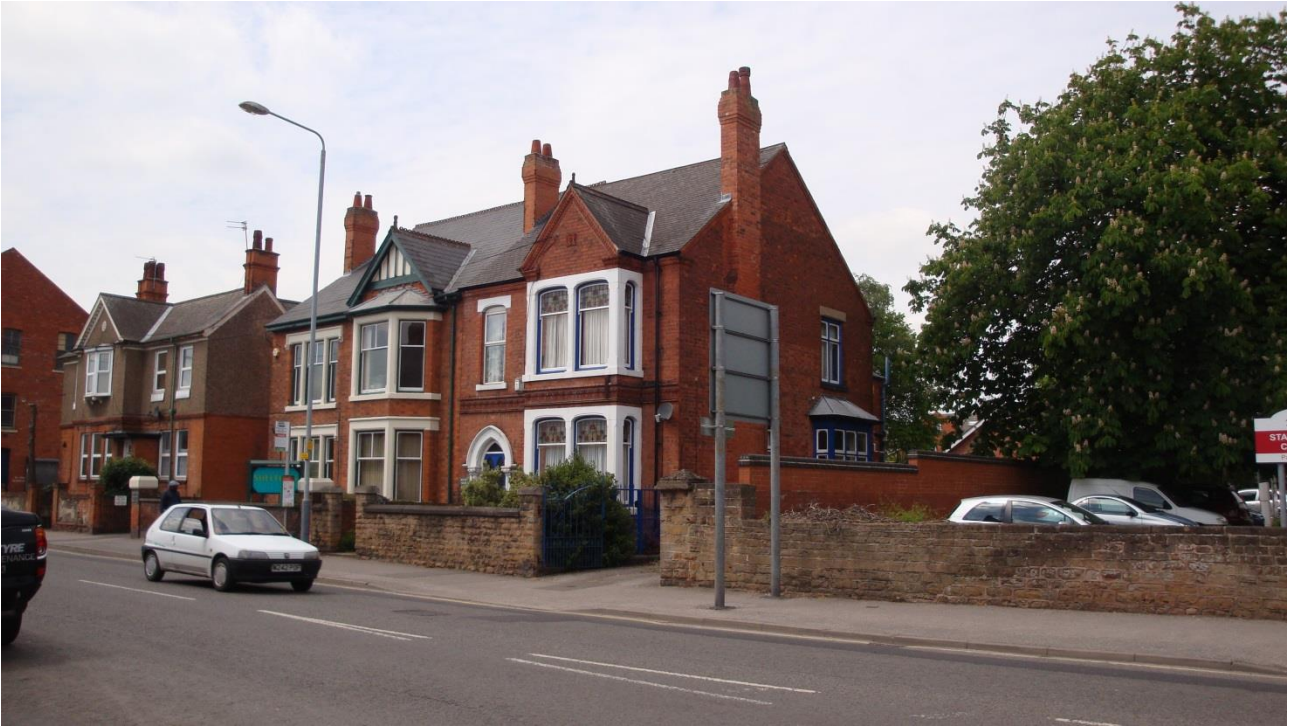
Figure B.9: North east façade of Rovert House, Station Street (Ref: 1329)
