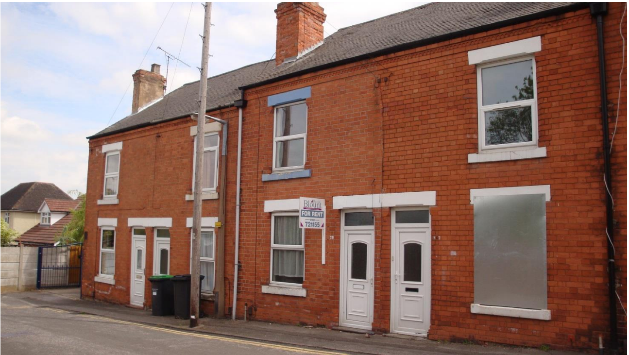
Figure B.1: West façade of 36 (on right of picture) and 38 Woollaton Street ( Ref: 1 and 1024) (No. 40 and 42 on left of picture)
