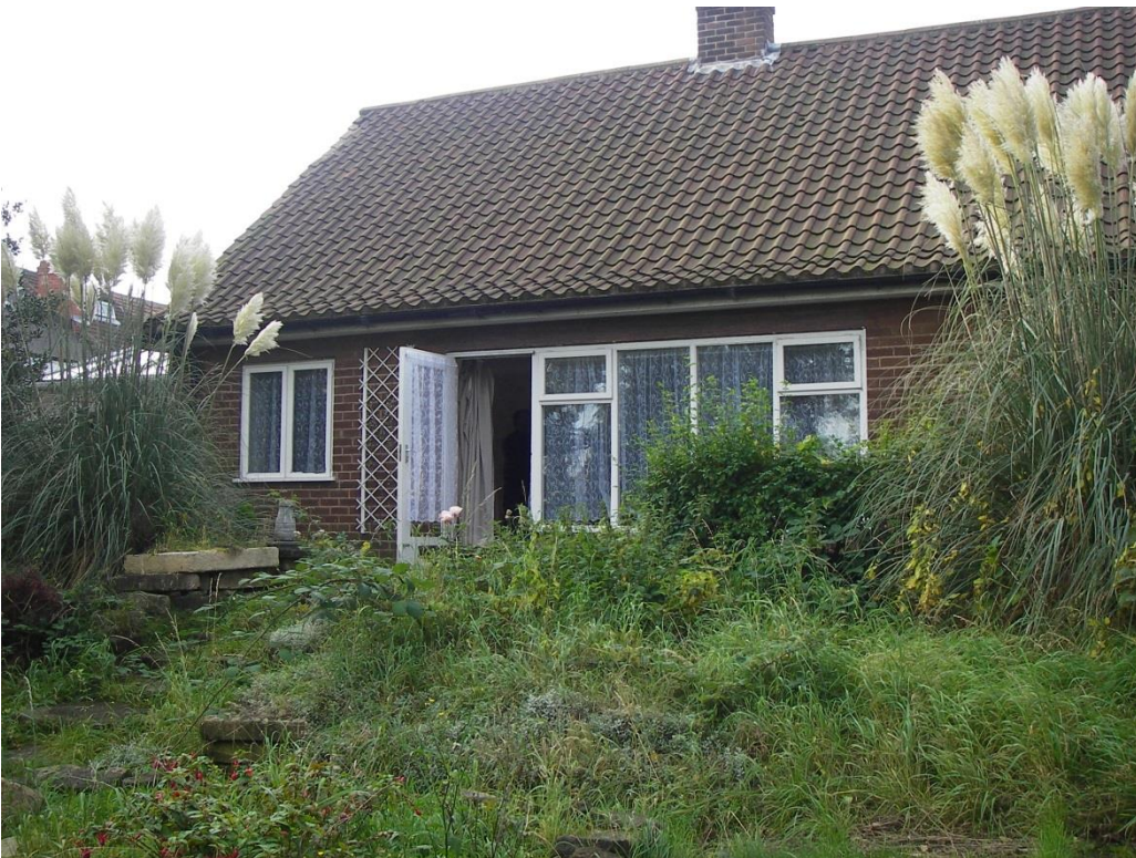
Figure B.12: North façade of 36a High Street (Ref: 1341), photo taken during 2008 baseline noise monitoring survey
