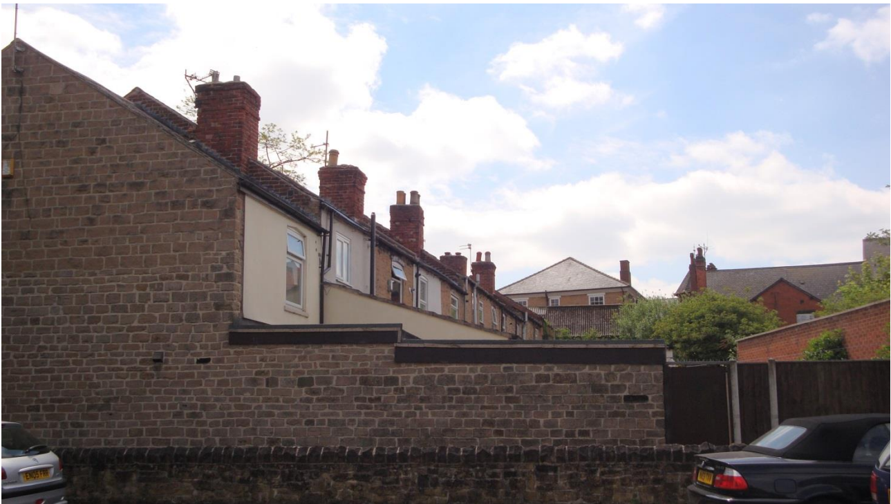
Figure B.14: North and west facade of 19 Albert Street (Ref: 1371)
