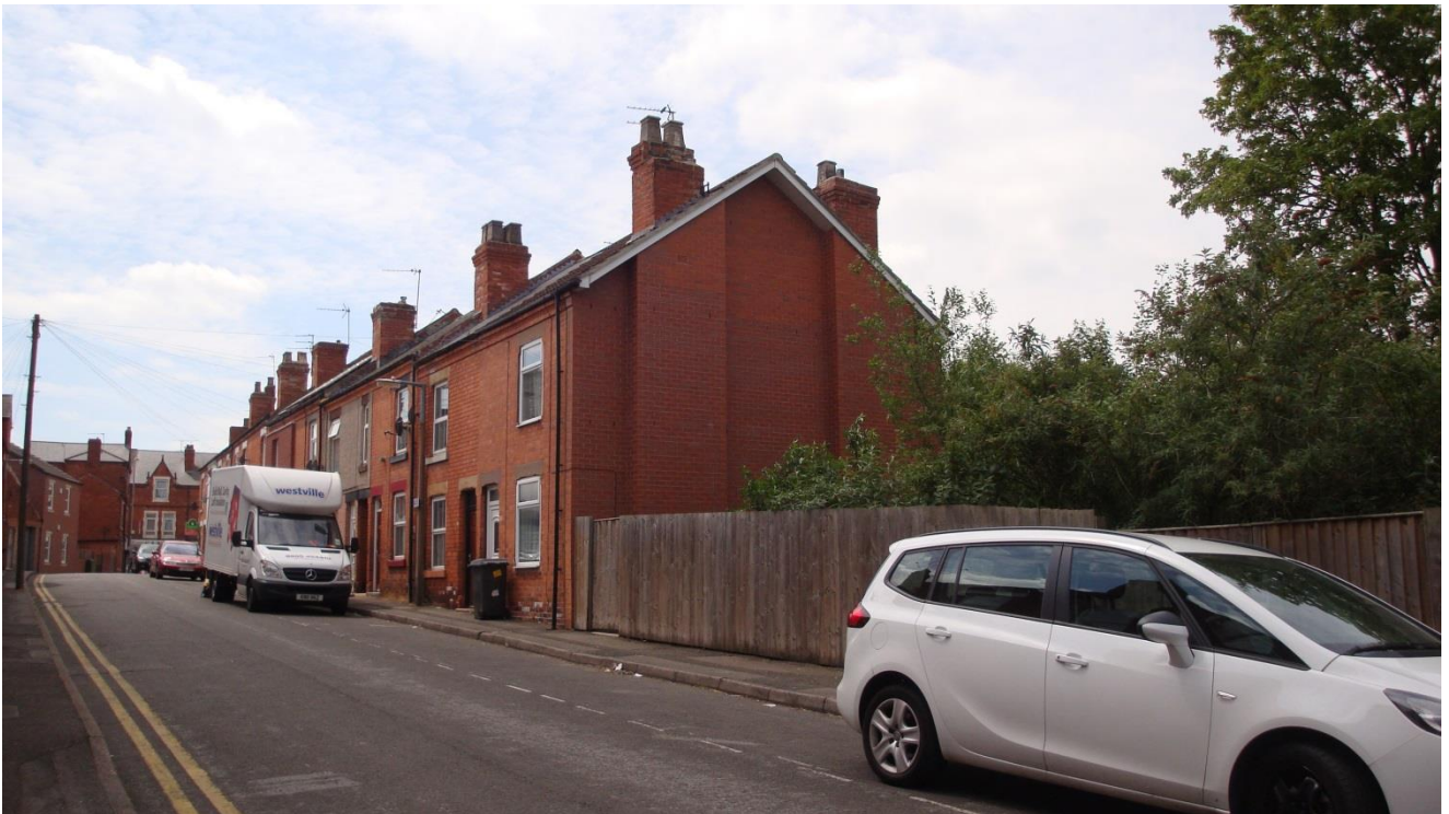
Figure B.4: East and north façade of 25 Woollaton Street (Ref: 5)
