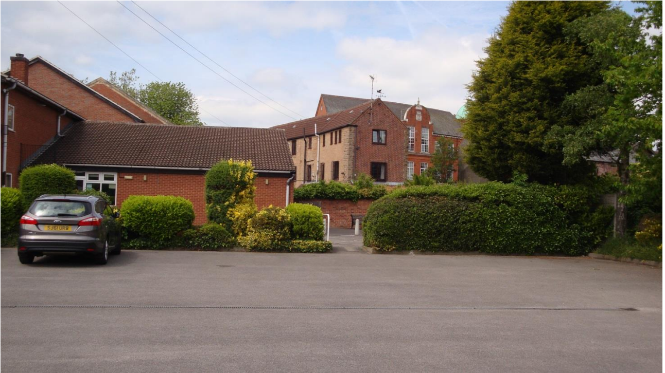
Figure B.7: East façade of 7 Wilcockson's Yard (Ref: 46) in centre of picture
