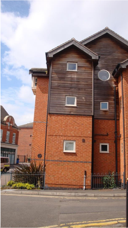
Figure B.5: East façade of Pinfold House (Ref: 122), only short section on left of picture qualifies under the Regulations, no windows or doors on this section
