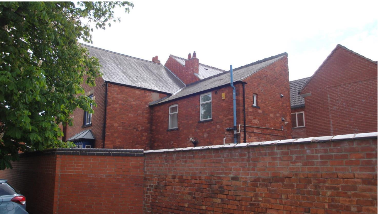
Figure B.10: North east and north west façades of Rovert House, Station Street (Ref: 1329)
