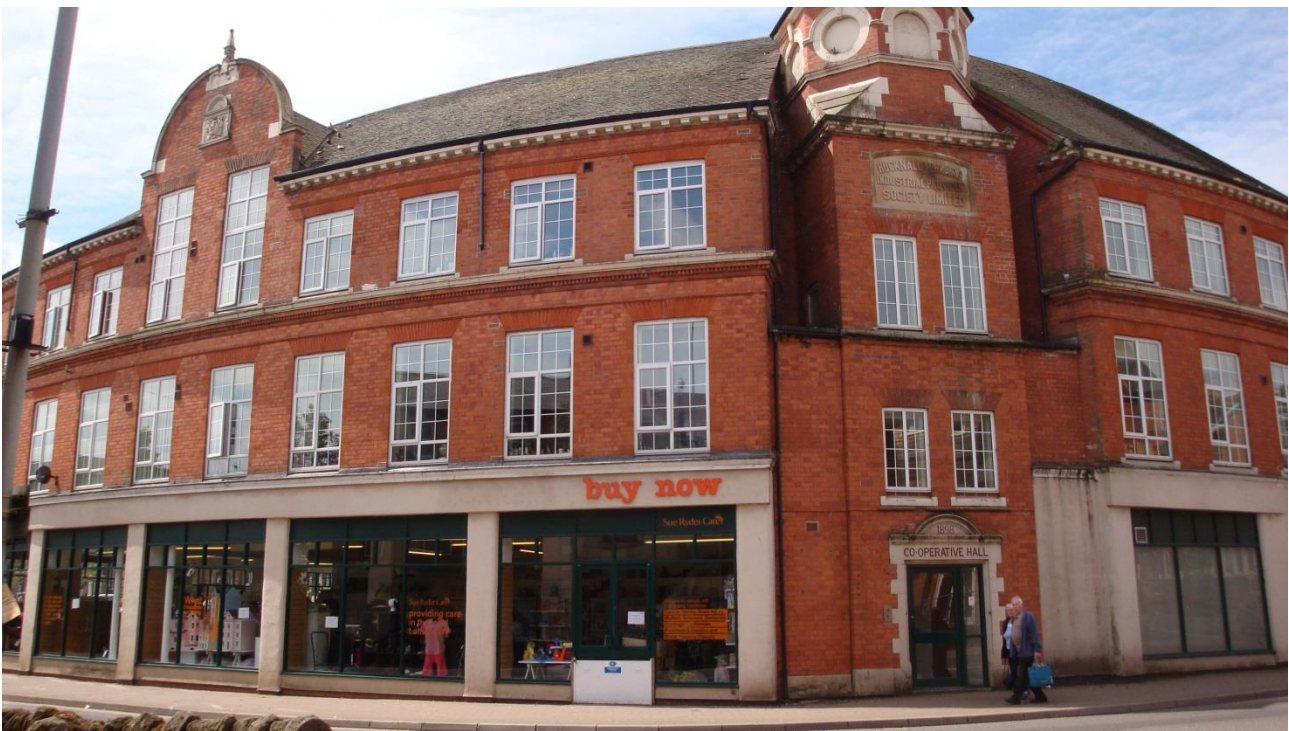
Figure B.18: East façade of The Byron Centre, corner of Baker Street and Annesley Road (Ref: 1789)
