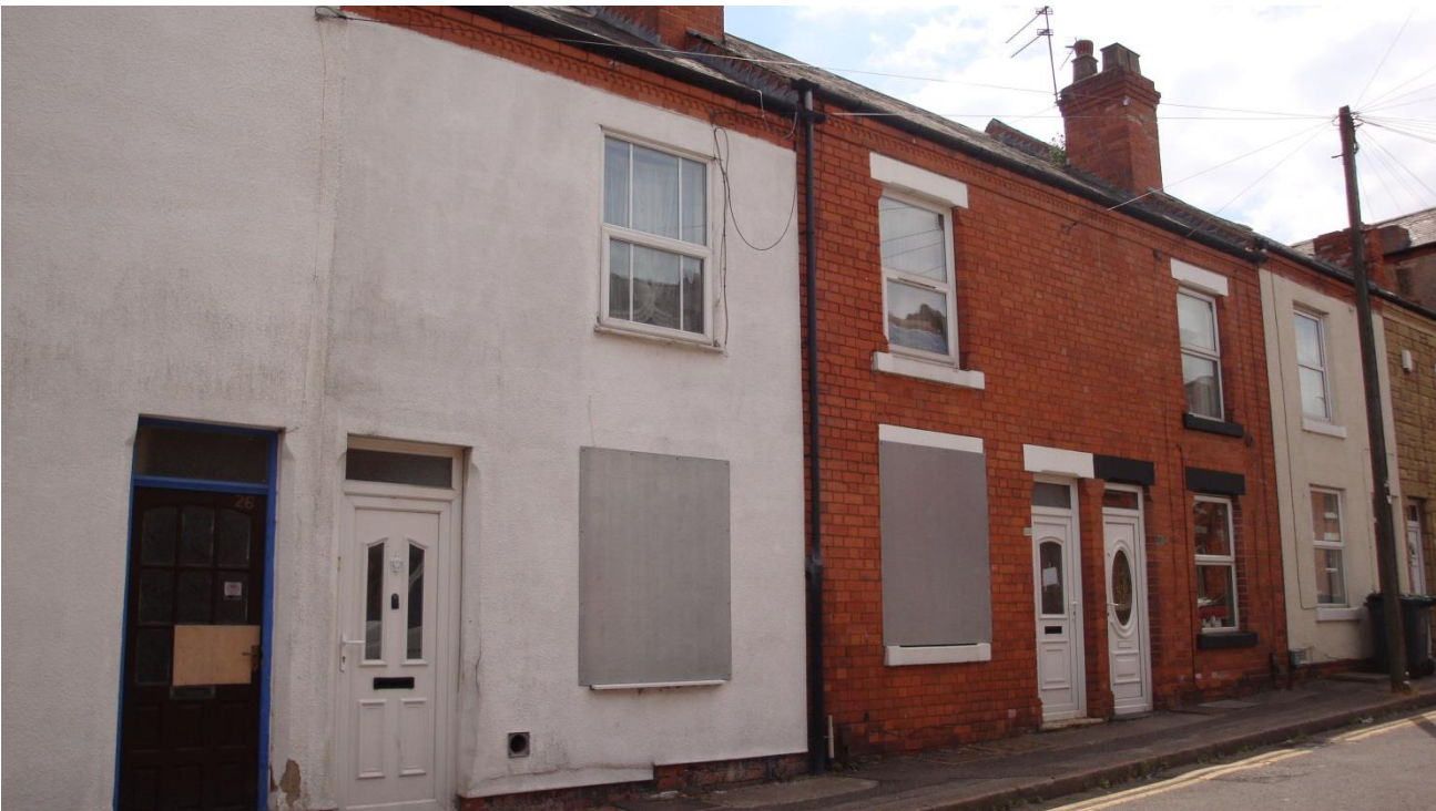
Figure B.2: West façade of 22 (in centre of picture) Woollaton Street (Ref: 2)
