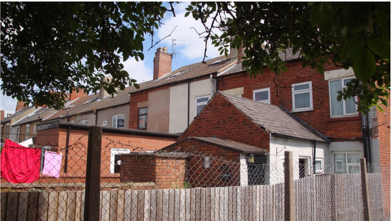
Figure B.16: West facade of 39, 41, 43 and 45 Albert Street (Ref: 1372, 1373, 1374 and 1375)
