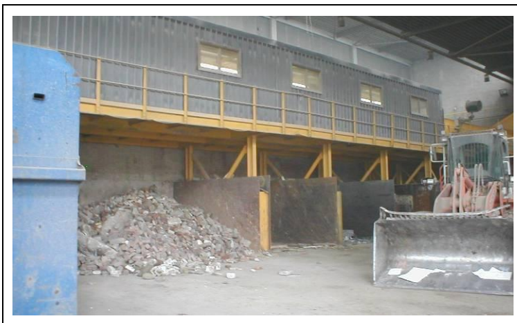
Figure A9.Site7.1: Indoor recycling hall.
