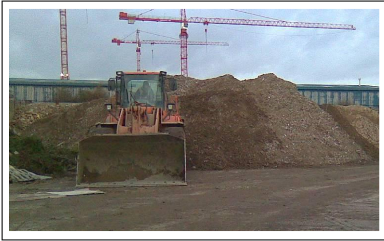
Figure A9.Site28.4: Stockpiles of soil and stones.
