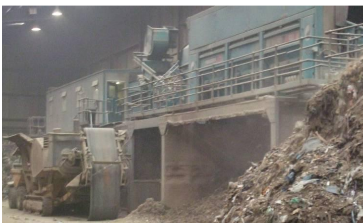
Figure A8.Site8.6: Older processing line and picking station.
