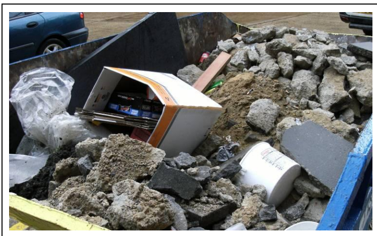
Figure A8.Site22.1: One of Site 22's skips adjacent to a small construction site, showing basically clean inert waste 'spoiled' by the presence of other wastes, both CDEW and other.
