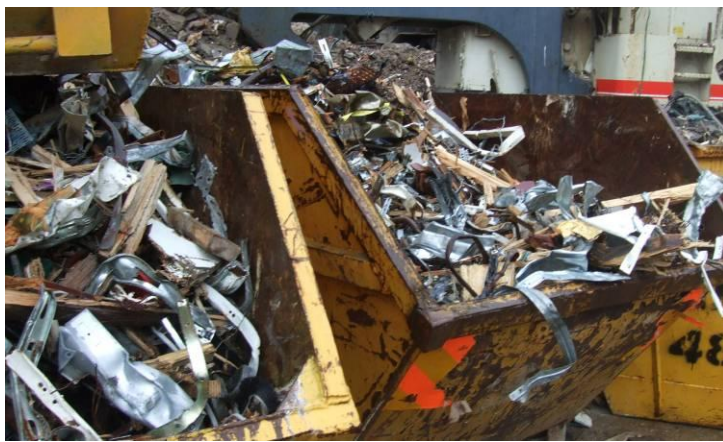
Figure A9.Site27.6: Mixed contaminants screened out of soil and hardcore.
