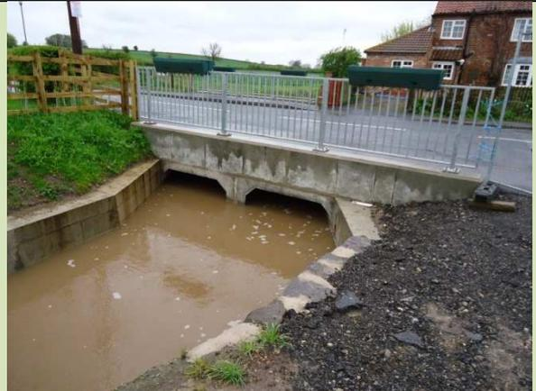
Photo 5.2: new culvert functioning during high flows
