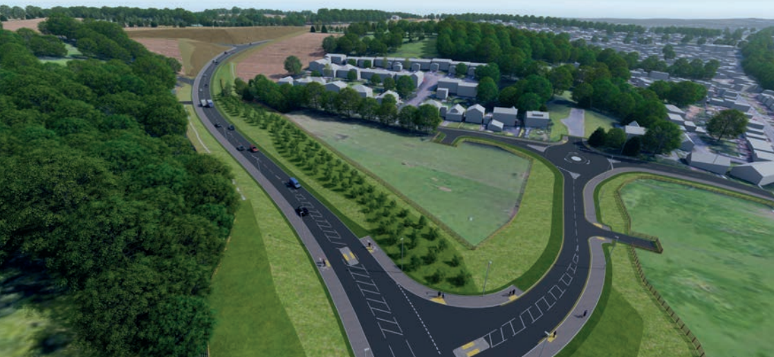
New Gedling Access Road
