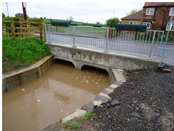
New Culvert in North Wheatley implemented through partnership funding, 2011
