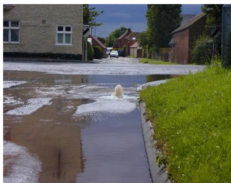
Surcharging drains in East Stoke (date unknown)
