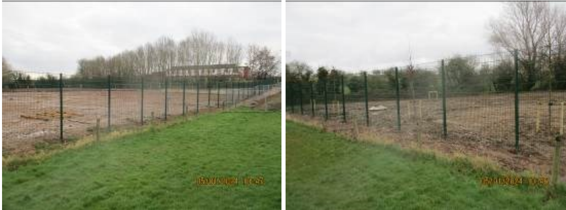
Left: Proposed playing field and retaining wall viewed from adjacent open space. Right: Trees planted adjacent to boundary fence.
