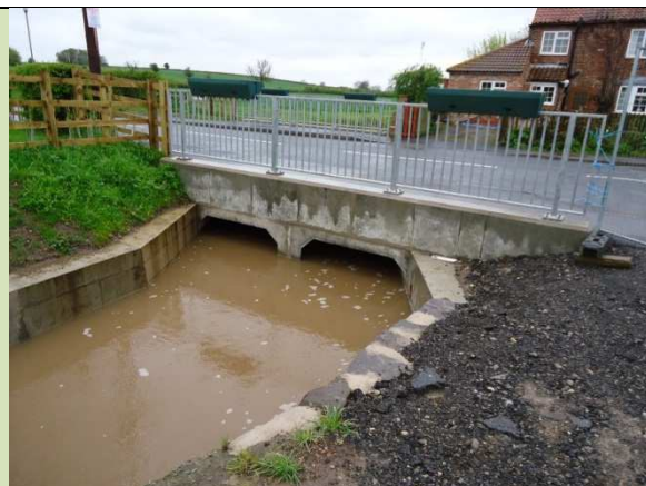
Photo 5.2: new culvert functioning during high flows
