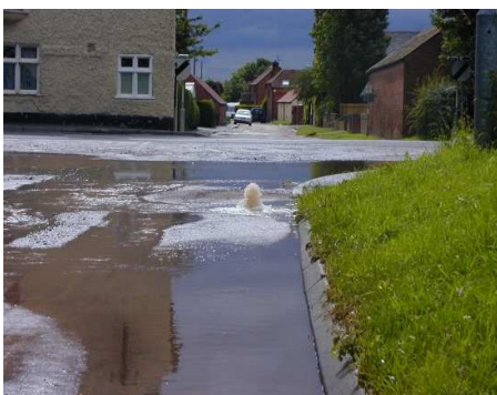
Surcharging drains in East Stoke (date unknown)
