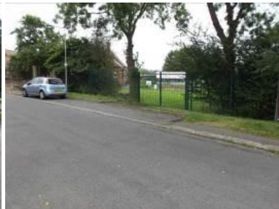
P2. Maintenance access gate – The Moor
