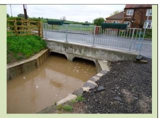
Photo 5.2: new culvert functioning during high
