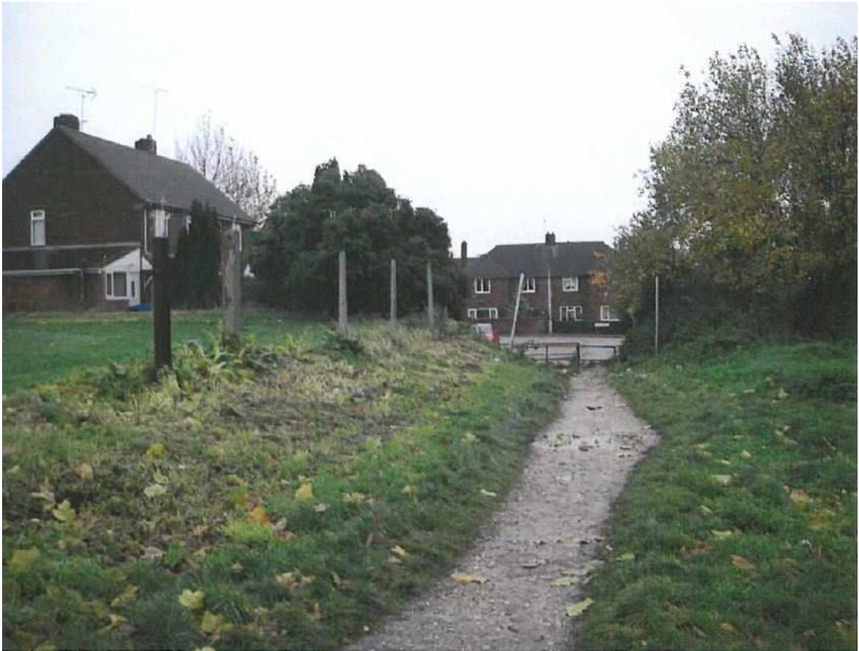
This undated photograph was taken by Bassetlaw District Council on route A-B-C looking towards the pedestrian access barriers at point 'C'.
