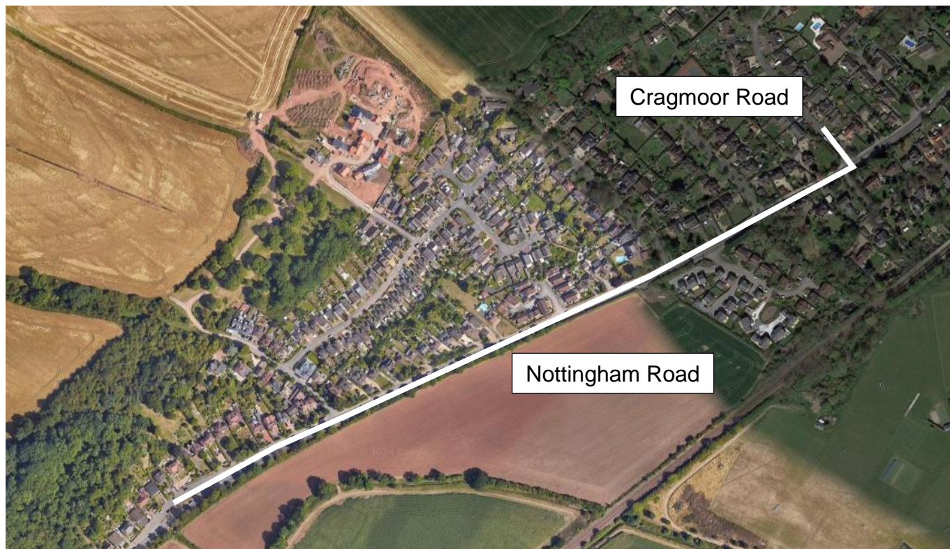
Figure 4. View of Nottingham Road and Cragmoor Road.
