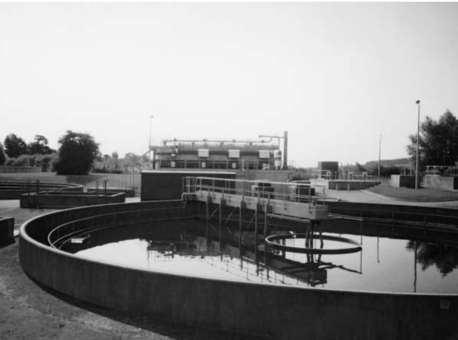
A typical sewage treatment works.
