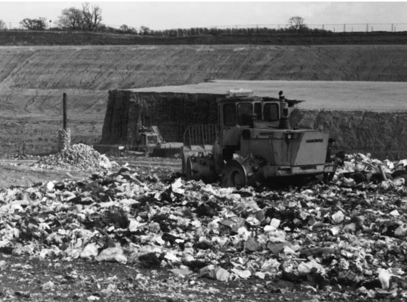
Dorket Head Clay Working and Landfill Site (near Arnold). Waste disposal will enable this mineral working to be reclaimed back to original ground levels.
