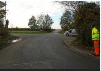
There is an existing footway on the north side of the A6097 from Gunthorpe to the signal junction and then a public footpath that connects to the A46 junction. The footpath looks well used. Pedestrians have no view of a left turning vehicle from the A6097, which could result in pedestrians stepping into the path of vehicles, with the potential for serious injuries to arise from any collisions that occur.
