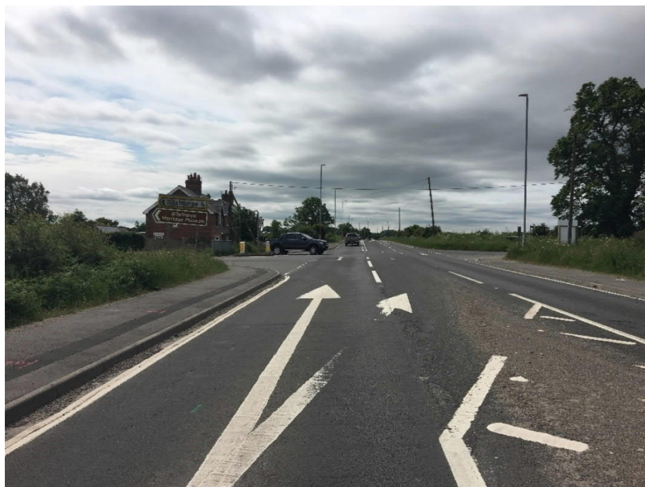
Plate 6-1 View to the south of Mickledale Lane Junction
