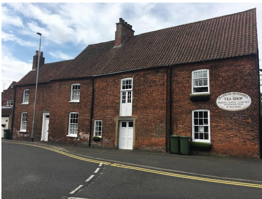
Plate 6-4 Ollerton Watermill and Mill House (1157098), north-east elevation
