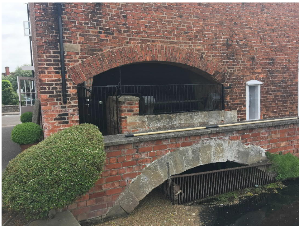
Plate 6-5 Ollerton water mill (1157098) south-west elevation, mill machinery details.
