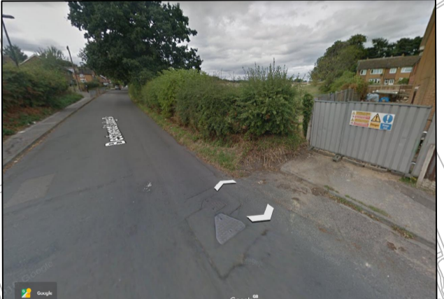
5. Bestwood Lodge Drive to be widened by 1.5m to allow bus access from the proposed new bus link.
