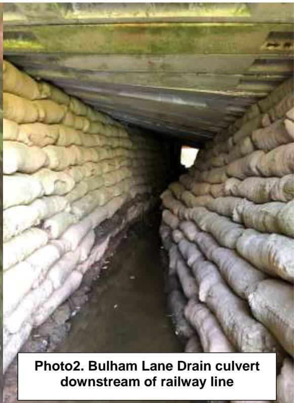
**Photo2. Bulham Lane Drain culvert downstream of railway line**
