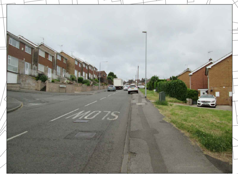
View looking south-west at steep gradient.
