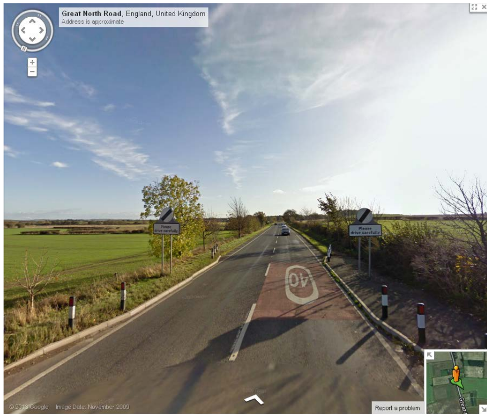
Figure 16 - Access Location - Barnby Moor
