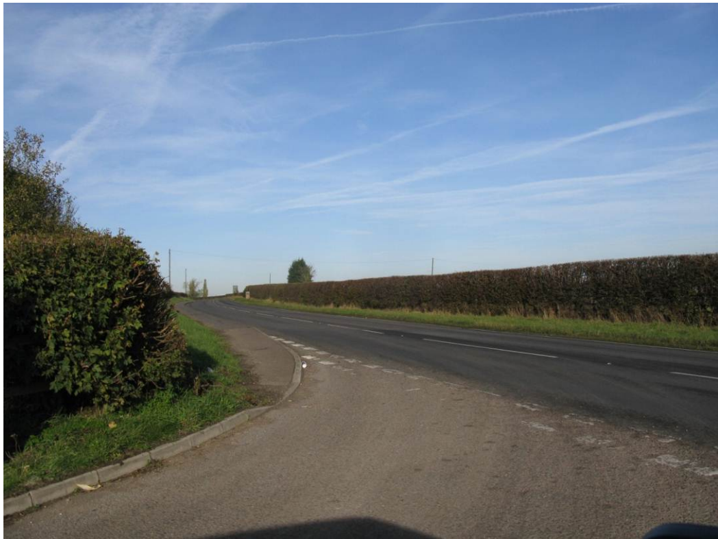
Figure 8 - Access Location - Besthorpe East
