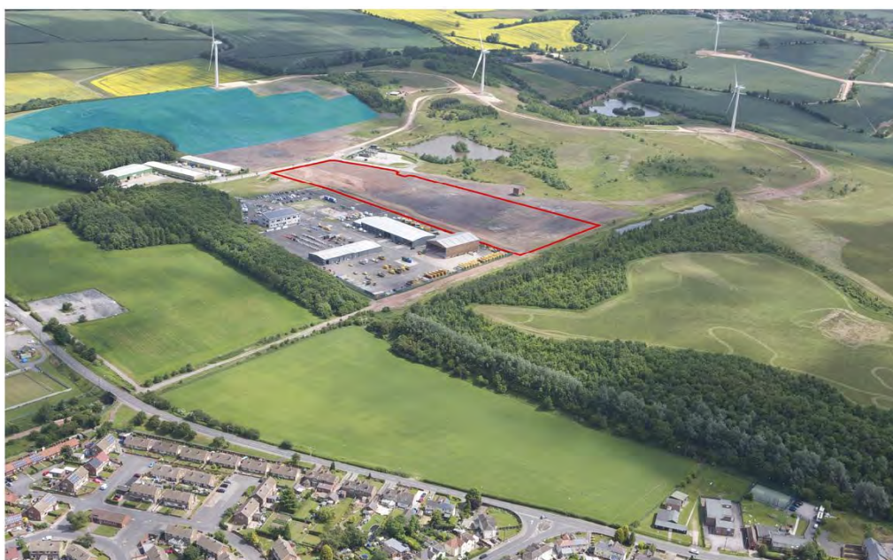
Photo 3.1: Mitigation area location
