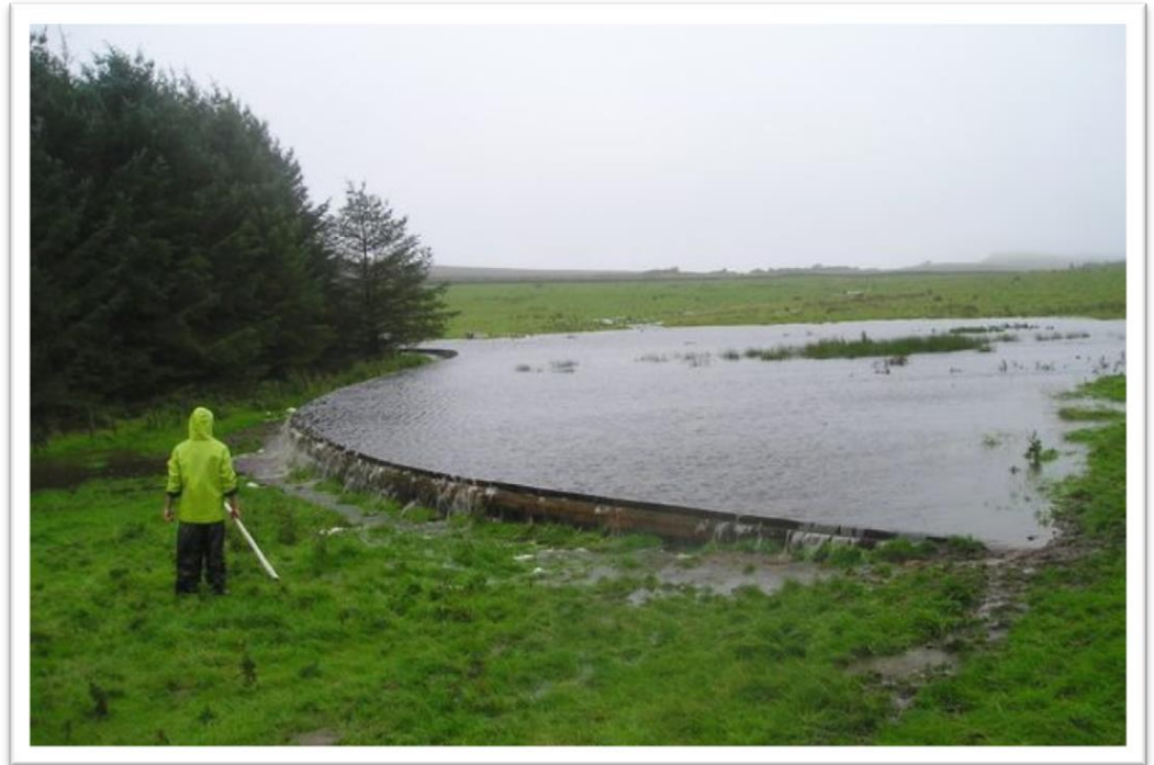
Informal Storage (Belford) Check weirs and/or control structures
