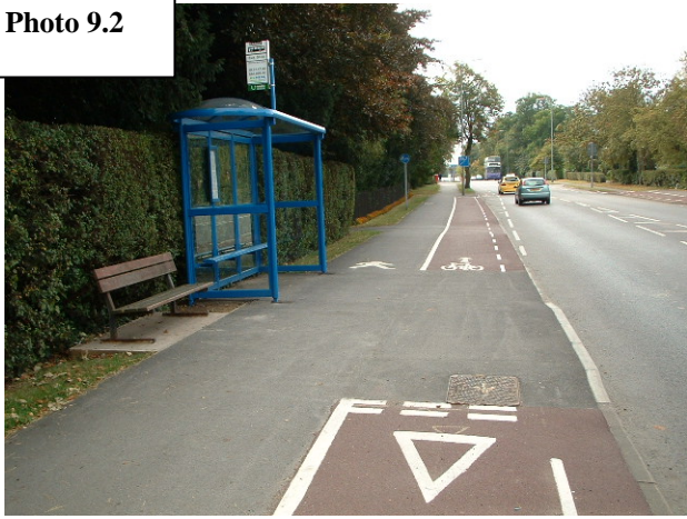
Photo 9.2 Cycle track gives way at bus stop. (Note: No tactile paving has been provided, however)
