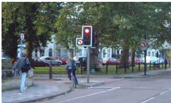
Photo 6.4 Cycle bypass at signal controlled junction. Courtesy CTC
