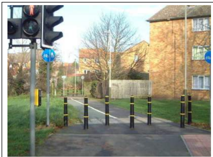
Photo 13.6 Staggered bollards make life more difficult for motorbikes but still allow for convenient access for cyclists, wheelchairs and pushchairs
