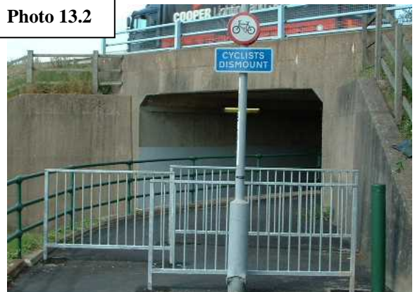
Photo 13.2 Shows a barrier layout that conforms to DfT Inclusive Mobility Guidance (Fig 13.A). Note that cyclists are instructed to dismount.
