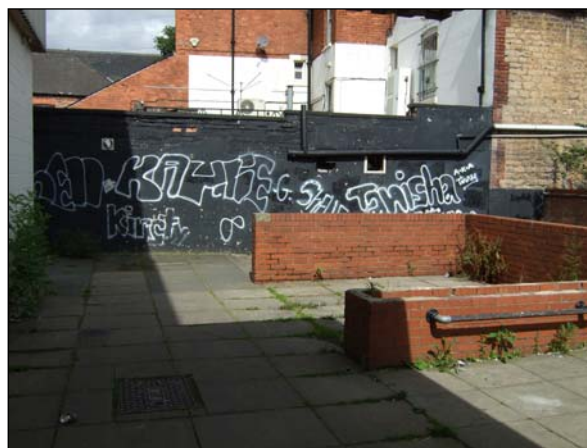
Photograph 11: Vandalism to the rear of the former Safeway building
