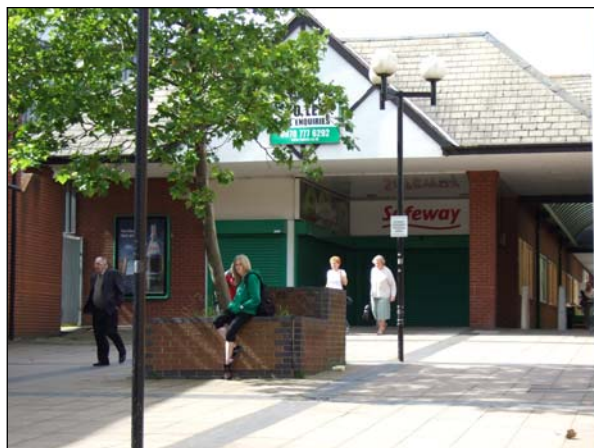
Photograph 10: Vacant former Safeway building
