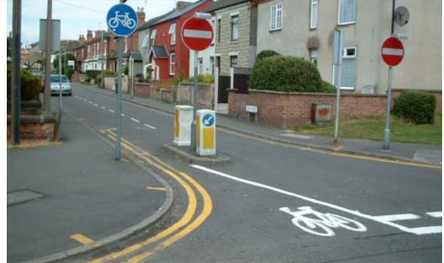
**Fig 4.D** No Cycle Lane (with segregation at entry and exit)
