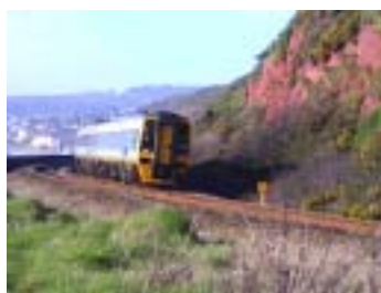
The railway between Teignmouth and Dawlish in Devon has been subject to landslips and cliff falls caused by coastal erosion, severing a main rail route.
