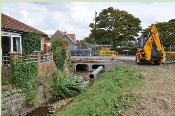
Photo 5.1: Construction in progress of new bridge flows and culvert
