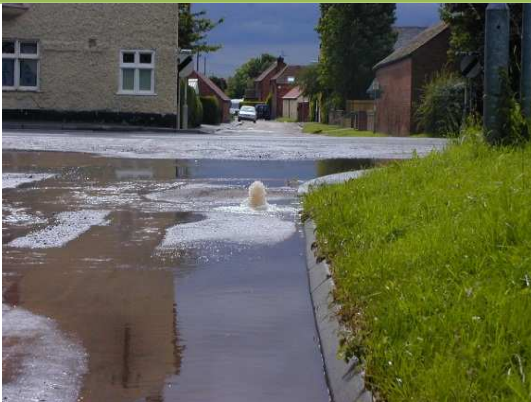
Photo 3.1.1: Surcharging drains in East Stoke (Source: Nottinghamshire County Council)
