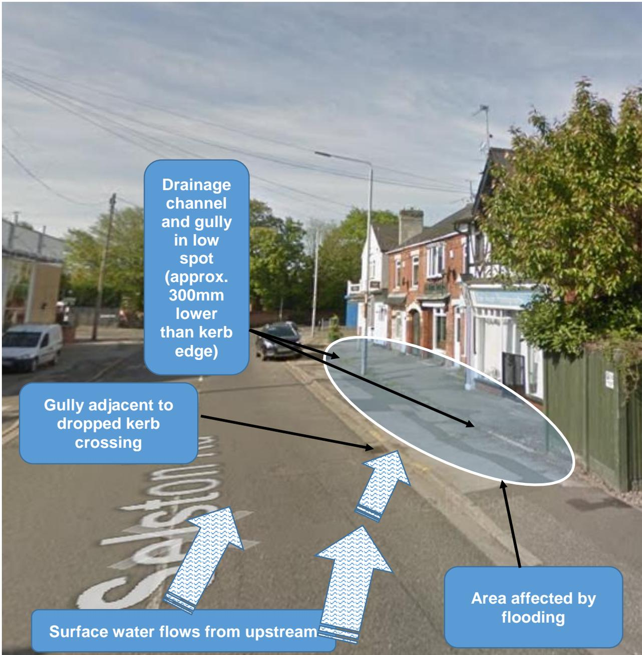
**Figure 6. Localised surface water flowpaths around affected properties**
