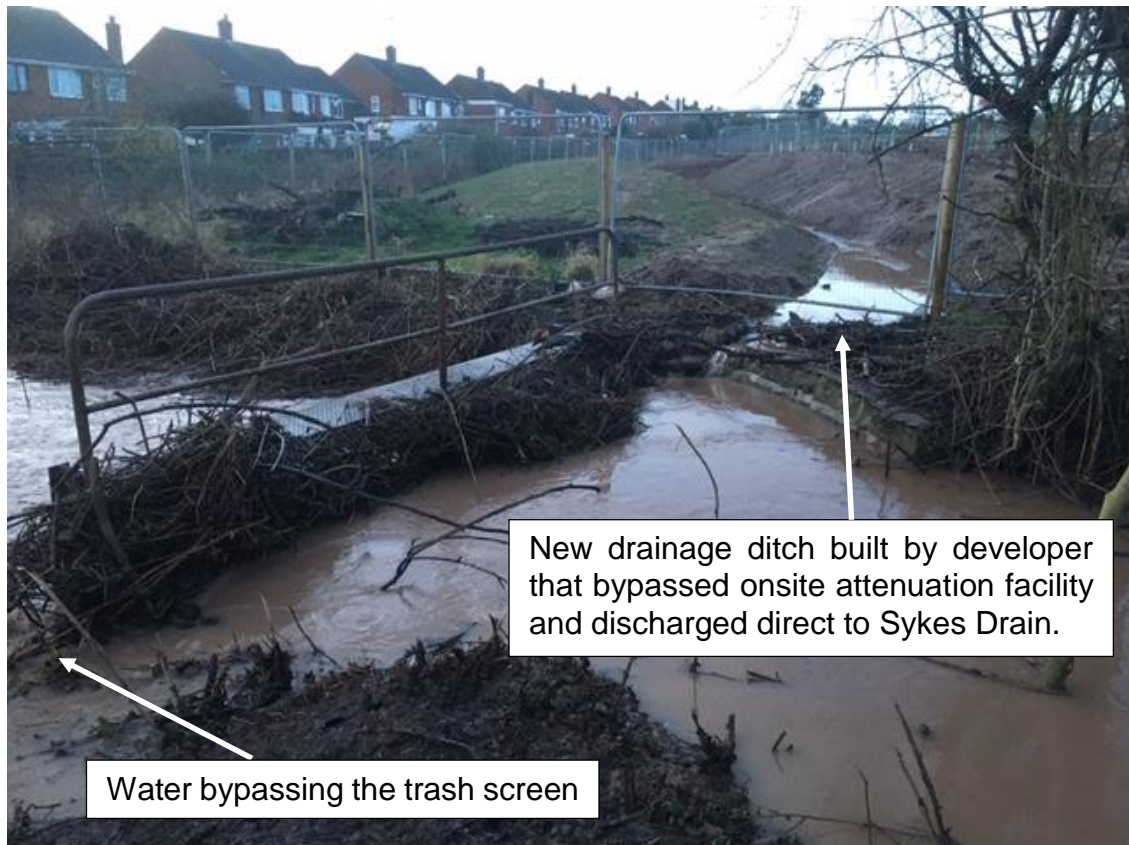
Photo 5. (Sunday 16 th February) showing the trash screen upstream of the culvert to be completely blocked to the extent that water is bypassing the screen on the left-hand side and the additional drainage ditch.
