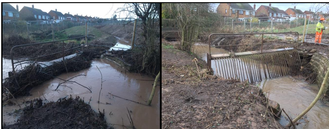
Photos 9. (left) and 10. (right) of the second trashscreen upstream of the mouth of culvert.
