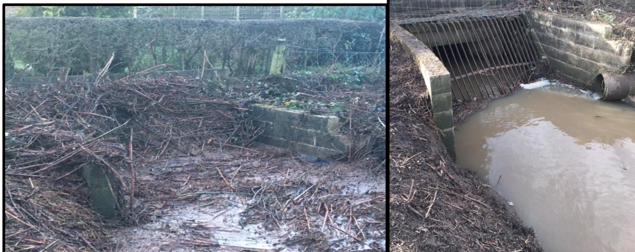
Photos 7. (left) and 8. (right) of the trashscreen on mouth of culvert.
