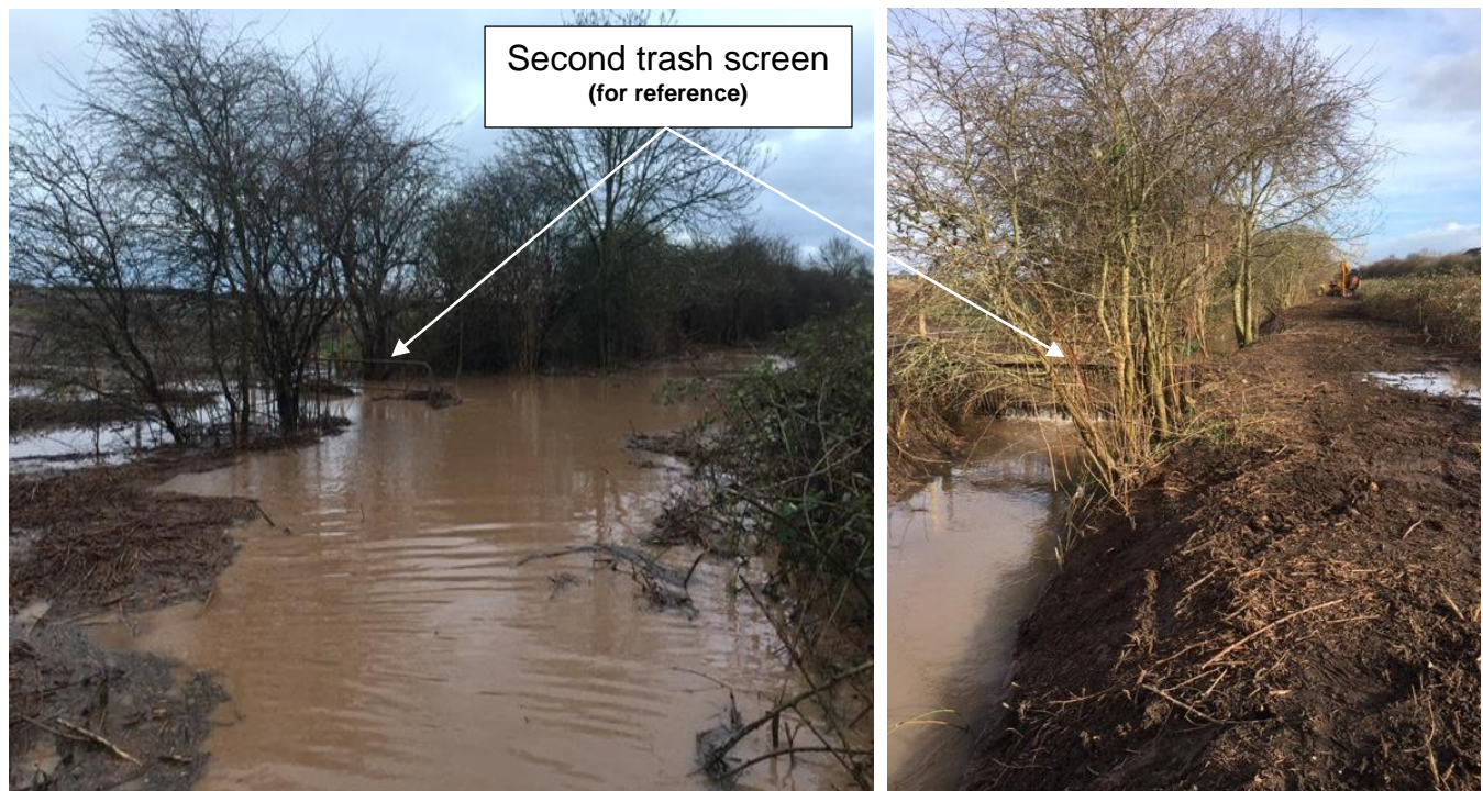
Photo 2. (left) Sykes Drain looking upstream from boundary of 87 Clumber Drive showing surcharge on Sunday 16 th February and Photo 3. (right) after trash screens and banks of watercourse cleared on Monday 17 th February.
