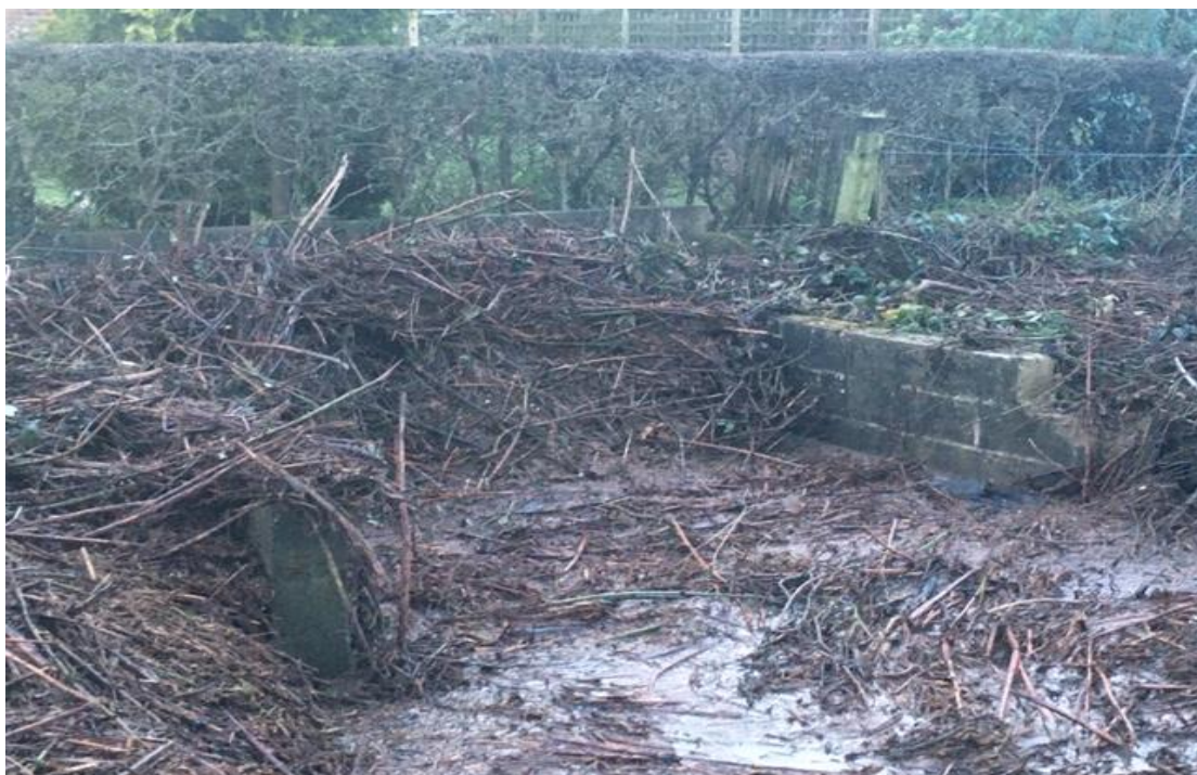
Photo 6. (Sunday 16 th February.) showing the debris blocking the trash screen on the mouth of the culvert. The trash screen is not visible due to the amount of debris.
