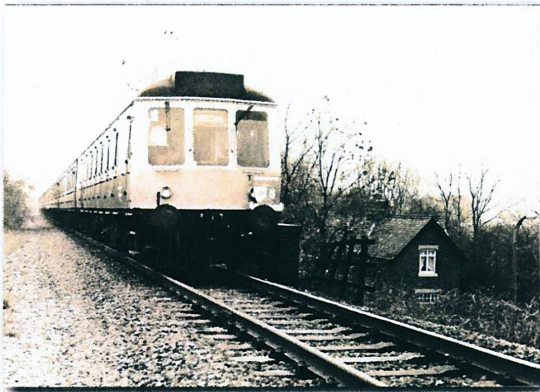
Diesel Multiple Unit on the bridge across Fackley Road in 1989. Note the station house to the lower right. ©Bill Taylor
