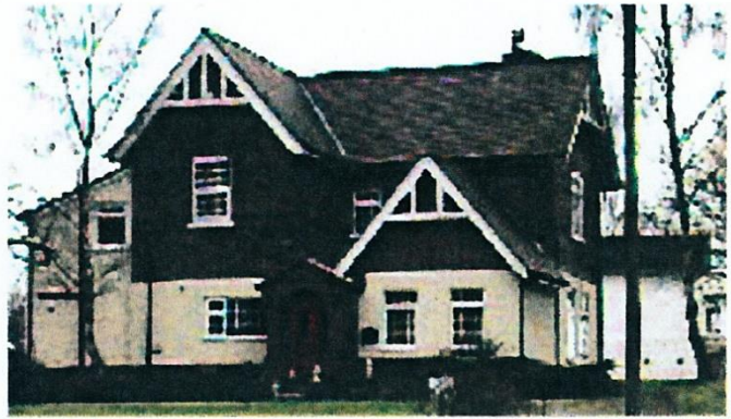
Teversal East Station Master's House
