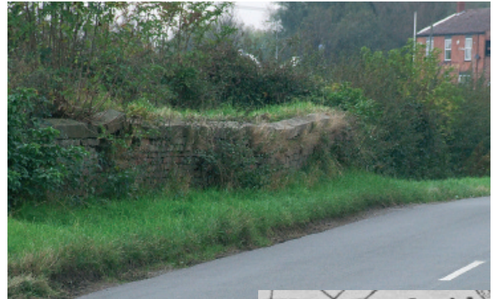
Site of the former bridge now
